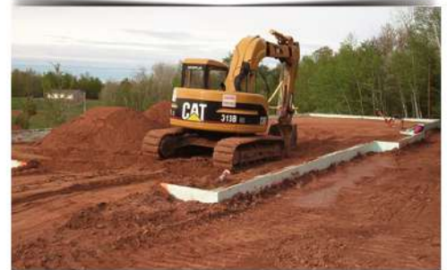
Back Filling works
